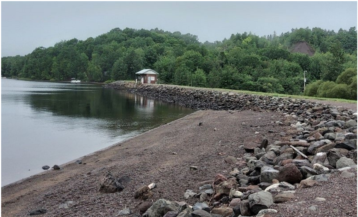
Photo 7: Unvegetated rip rap armored shoreline with beach-like foreground. View to southwest.
